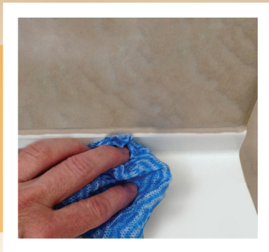
Dual Stage Tile Flange with Tile Installed
